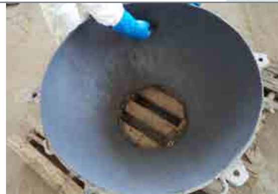
Application of ARC coatings.
