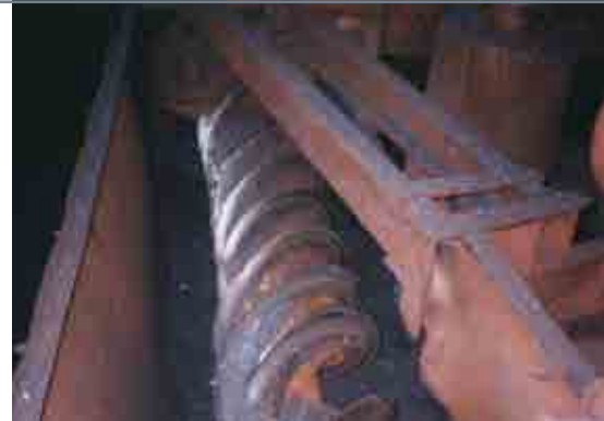
Old screw showing weld overlay repairs.
