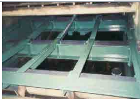
ARC BX2 applied to top rails
