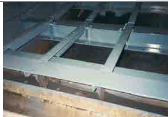
ARC S2 grey applied to coal screen
