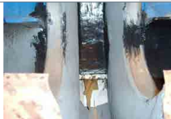
Pumps rebuilt with ARC 858 and ARC MX2 . Top coated with ARC 855 .
